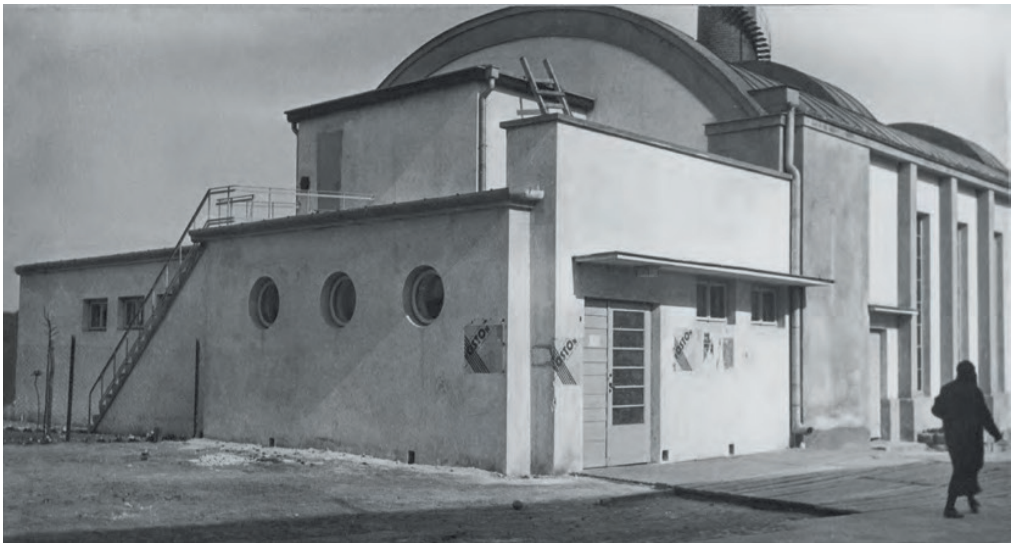
Central boiler station building at the Warsaw Housing Cooperative (WSM) estate, Żoliborz, Warsaw, visible poster for the show Boston (1934), WSM Hall of History
