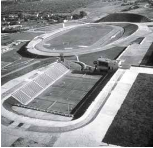
A 'bulge-and-hollow' at the Warszawaianka sports complex — a sunk tennis-court area with wind-breaker earth banks, 1965; photo: Zbyszko Siemaszko / Polska Agencja Fotografów FORUM
